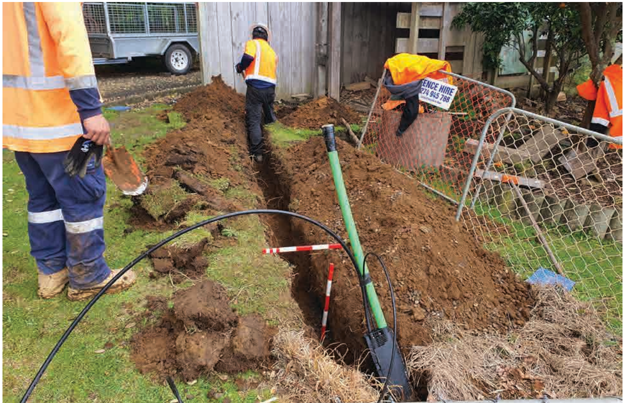
Figure 4. View south of trench outside 47 Ngakoti Street.
