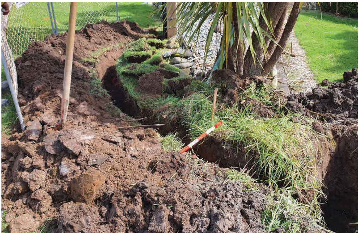
Figure 5. View west of trench outside 51 Ngakoti Street.
